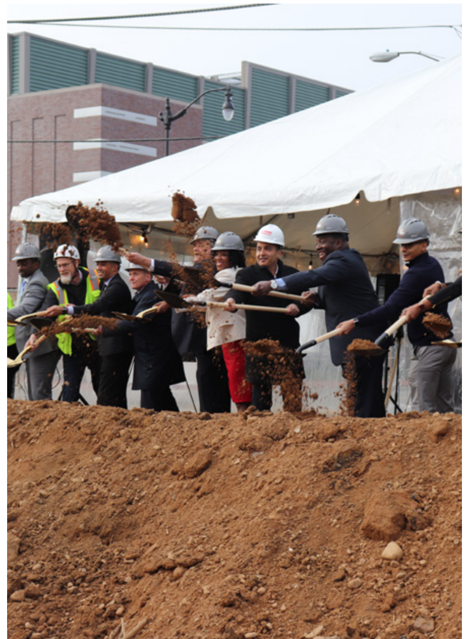
UPO President and CEO Andrea Thomas (in white) at the groundbreaking
